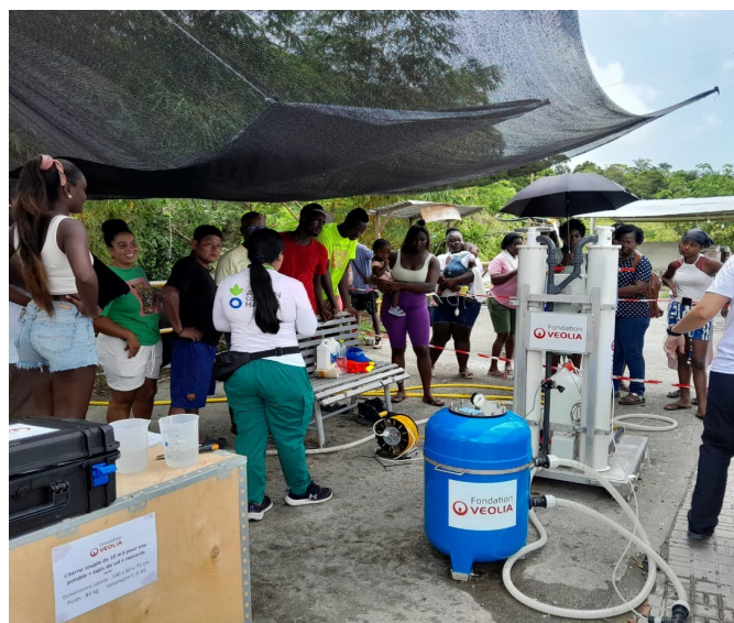
Installation and commissioning of the water treatment plant in San Rafael El Dos, Unión Panamericana, 28/08/2026
